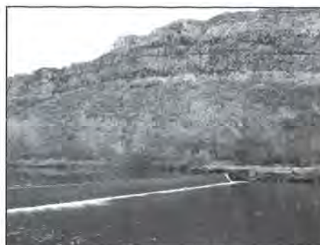
This irrigation diversion on the Cache la Poudre River in Colorado is an example of a low-head dam (WWE).
