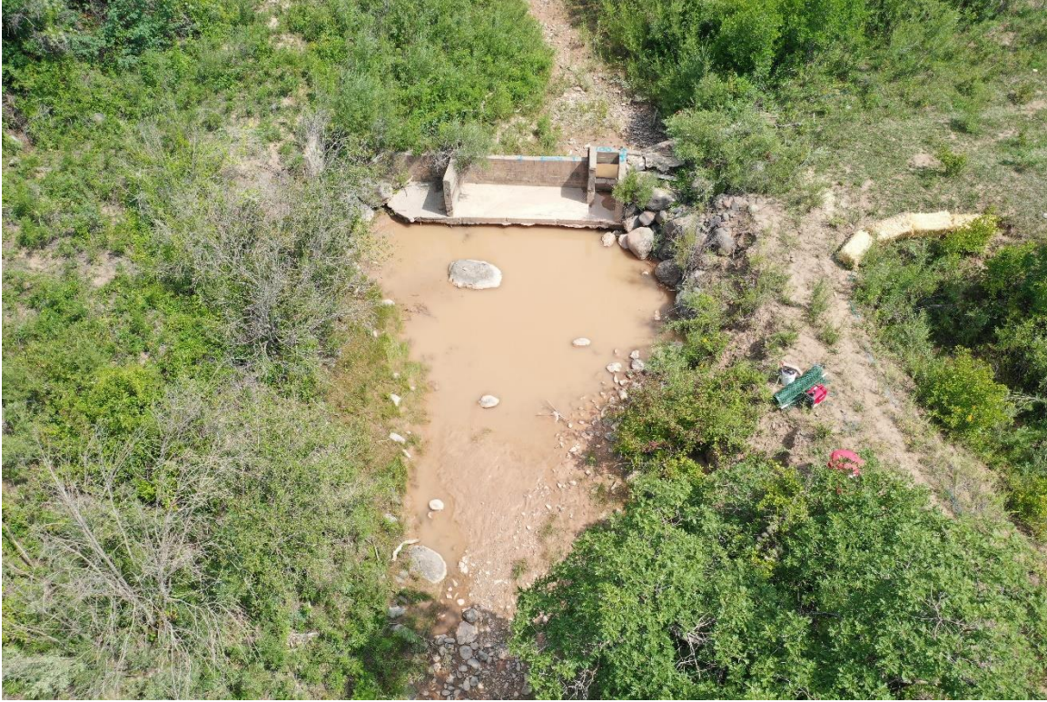
Aerial view before construction (August 2021). Photo credit Scott Schreiber, Wright Water Engineers.
