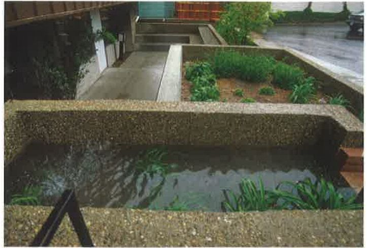
Figure 8. Detention pond on western side of ECR building receiving runoff from the building’s roof. The pond empties into a xeriscape planter. Date: approximately 1998.
