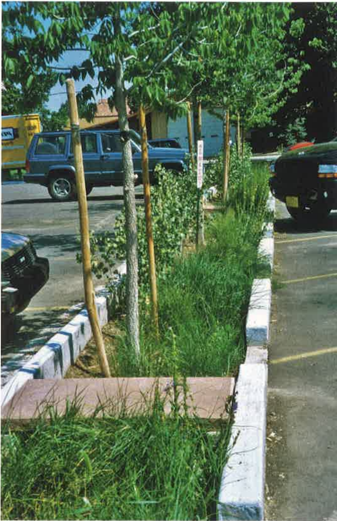
Figure 3a. Parking area landscape buffer with shade trees and native species shortly after installation in 1998. The image shows positive drainage into the buffer area from the surrounding paved parking spaces.
