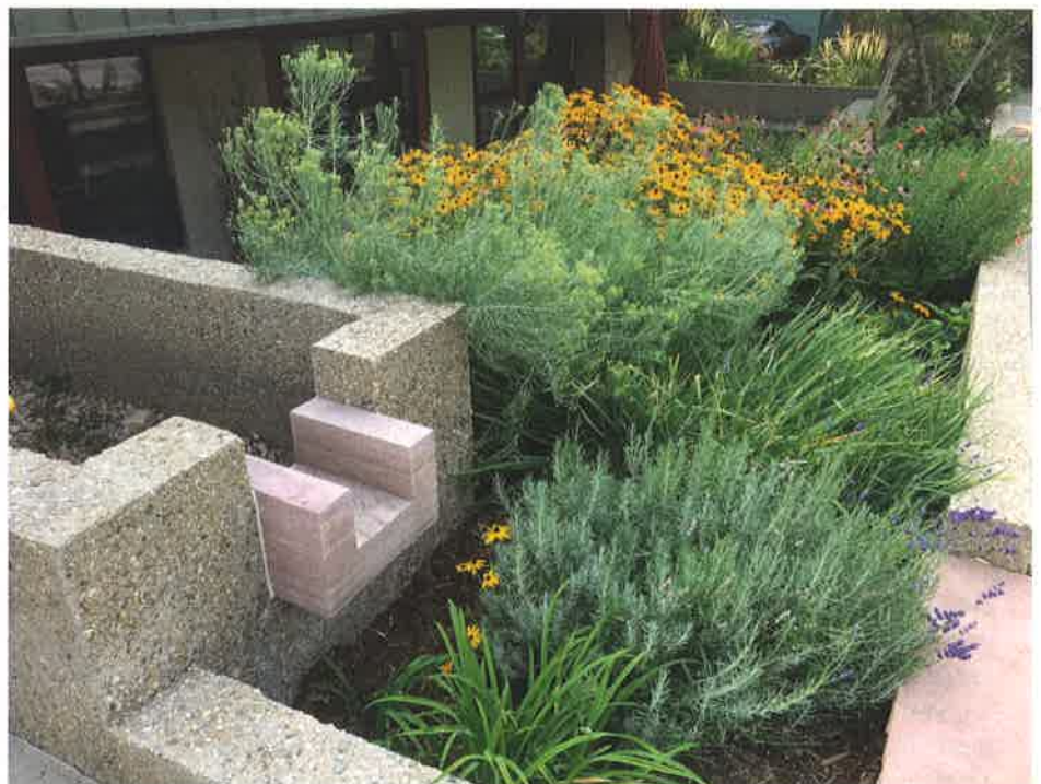
Figure 9. Infiltration gallery with a xeriscape planter on western side of building promotes runoff detention and infiltration. Date: 2017.
