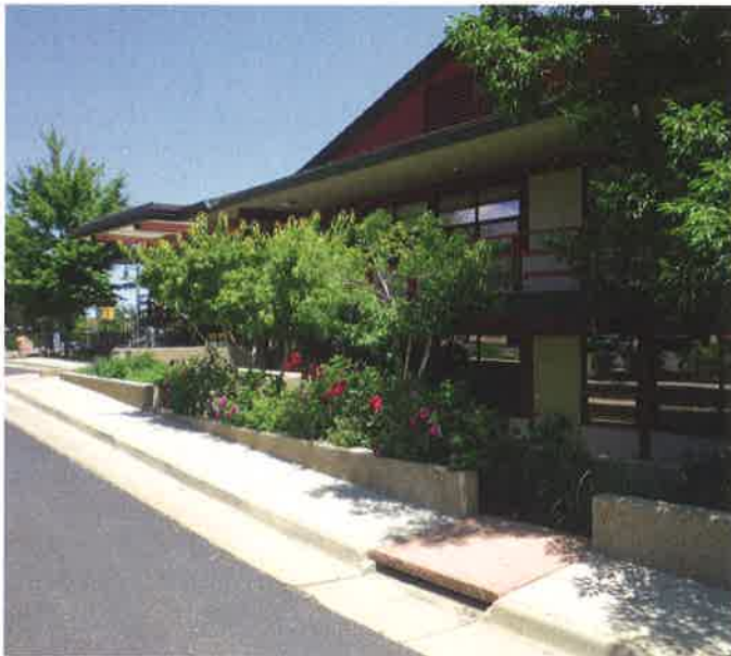
Figure 10. A series of interconnected planters on the building's west side collects and infiltrates roof and parking lot runoff. They have been planted with xeric ornamental plants and trees to shade the outdoor amphitheater and building from hot afternoon sun at the main building entry. These are in contrast to the native plantings that were used in the 1998 landscape renovation along the north and east building edges. Date: approximately 2008.
