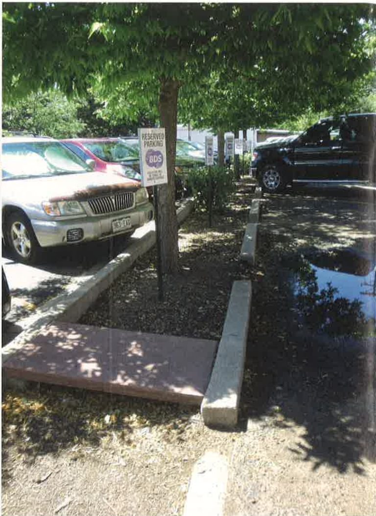
Figure 3b. Parking area landscape buffer in 2017. Sediment has filled the landscape buffer, and mature woody plants prohibit sediment removal.
