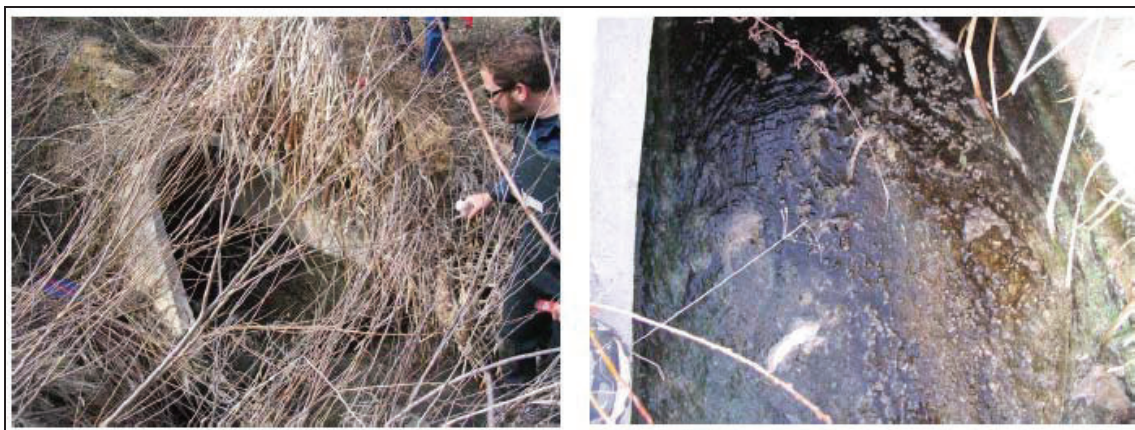
Photos 1 and 2. A dry weather sanitary survey resulted in identification of an illicit discharge to the storm sewer due to a plumbing error at a residential home. Toilet paper, odor, elevated temperature and other factors lead to identification and removal of this discharge.
