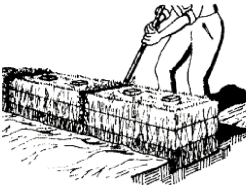
3. Wedge loose straw between bales.
