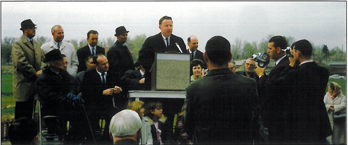
Mayor Currihan dedicates the Harvard Gulch Flood Control Project in 1967.
