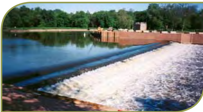
Figure 7. Island Farm Weir stepped spillway modification.
