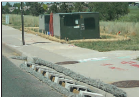
Silt fence and undisturbed vegetative buffers, right, serve as perimeter controls for non-potable water pipe installation. Straw wattle perimeter control and inlet protection safeguard water quality during underground electrical construction.
