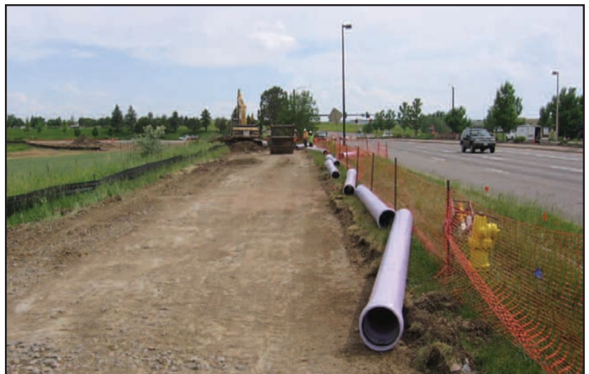
Silt fence and undisturbed vegetative buffers, right, serve as perimeter controls for non-potable water pipe installation. Straw wattle perimeter control and inlet protection safeguard water quality during underground electrical construction.
