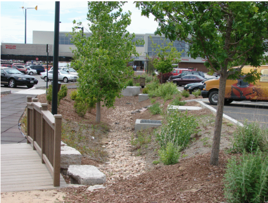
Photograph 3. Bioswale at Wal-Mart, Tower Road and Interstate 70, Aurora, Colorado
