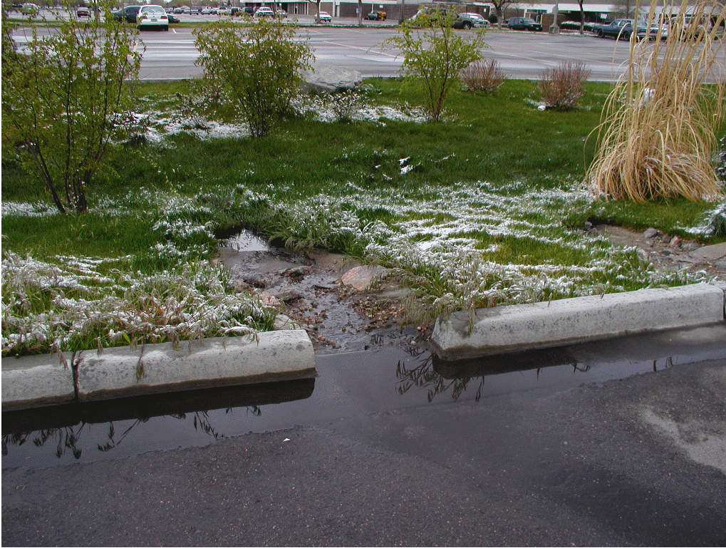
Photograph 2. Bioretention/Porous Landscape Detention, Aurora, Colorado
