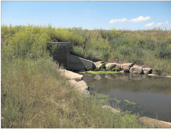
**Fig. 5.** Pond W-6/W-7 outlet and micropool
